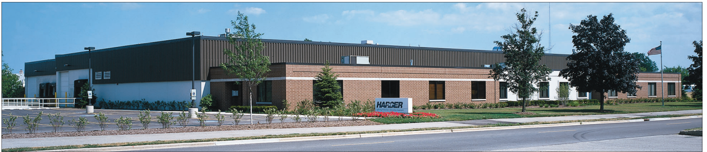
Harger's corporate office and 66,000 square foot manufacturing facility located in Grayslake, IL.
