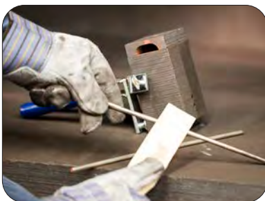
Step 2: Clean and dry conductors, insert conductor into mold, close handle clamp and lock mold.
