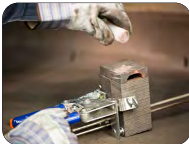
Step 5: Close lid, remove Orange cap from starting powder chamber and sprinkle next to ignition hole.
