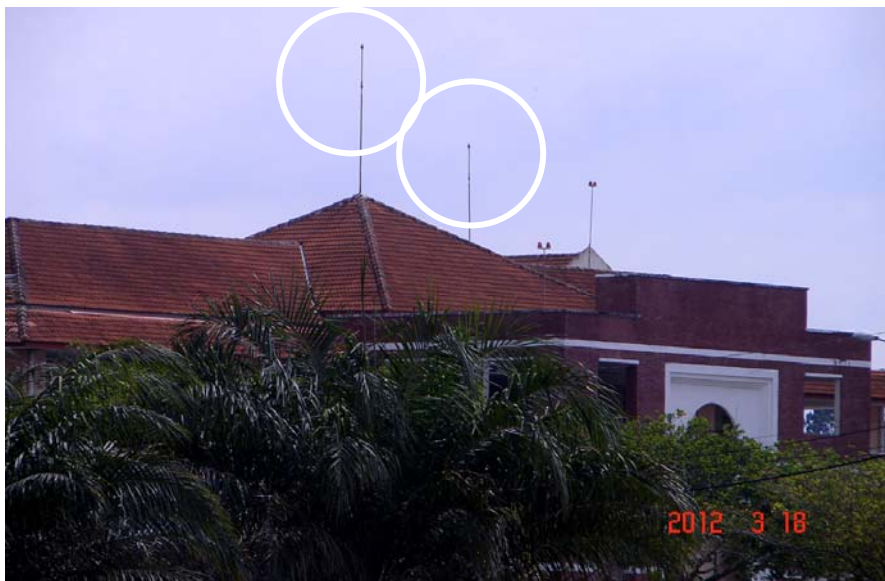
Fig. 2: Another KUIM building with the ESE lightning rods.
