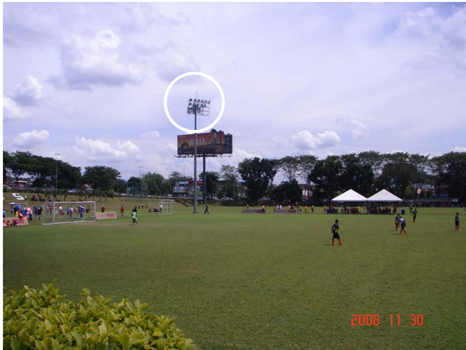
Fig. 15: An ESE lightning rod installed on the floodlight of a football field.
