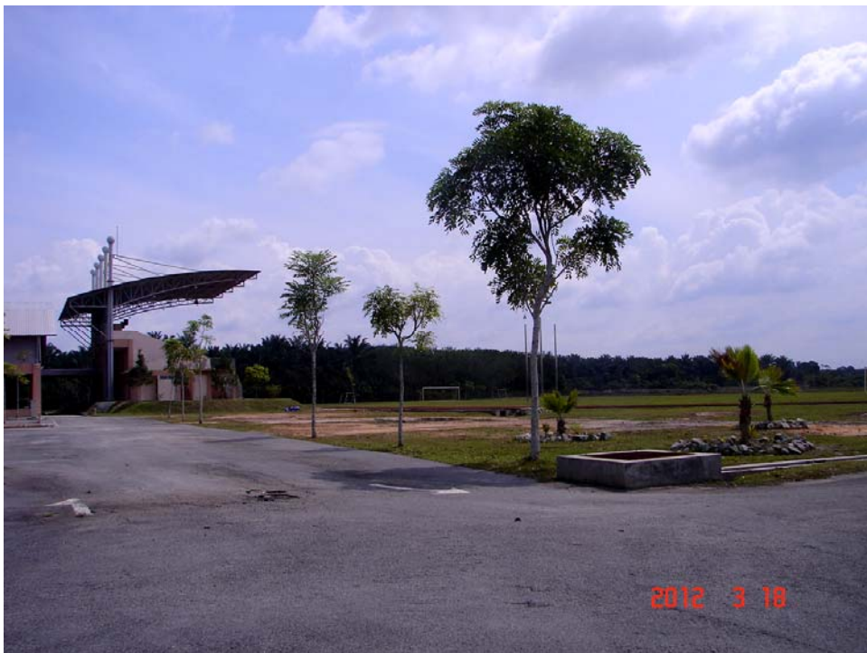
Fig. 4: Side view of the grandstand and football field.
