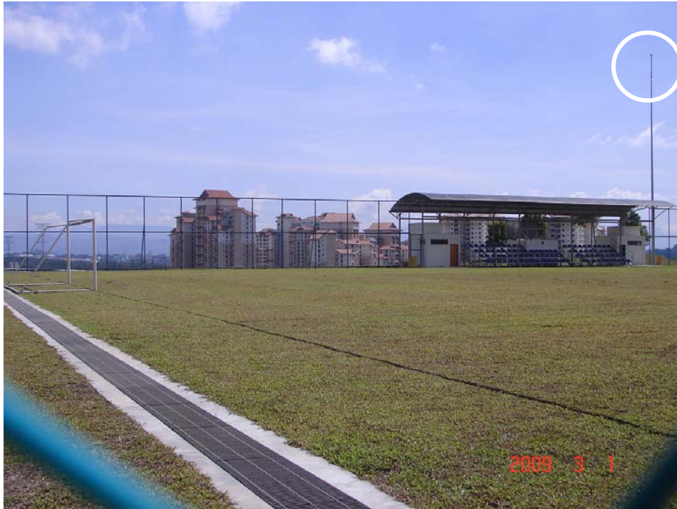
Fig. 13: An ESE lightning rod installed on a school field in Putrajaya.
