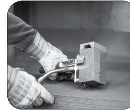
Step 1: Dry and clean the mold and conductor.
