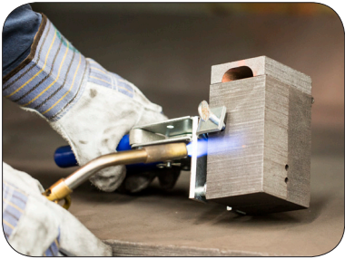
Step 1: Dry and clean the mold and conductor.
